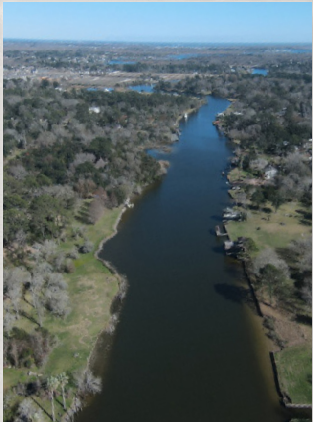
Dickinson Bayou facing east at Union Pacific railroad bridge Source: Halff Associates
