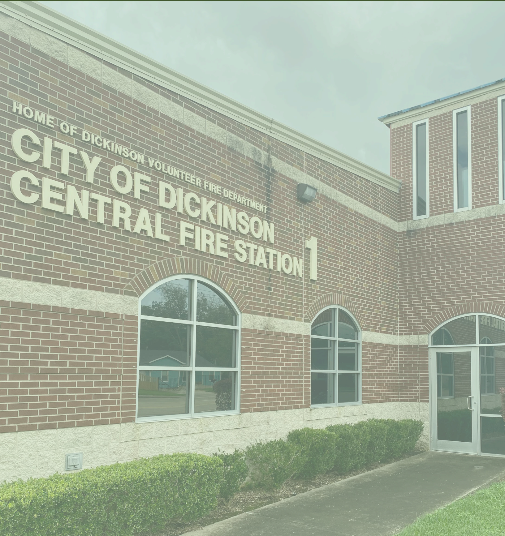
Dickinson Volunteer Fire Department Central Fire Station #1 Source: Halff Associates
