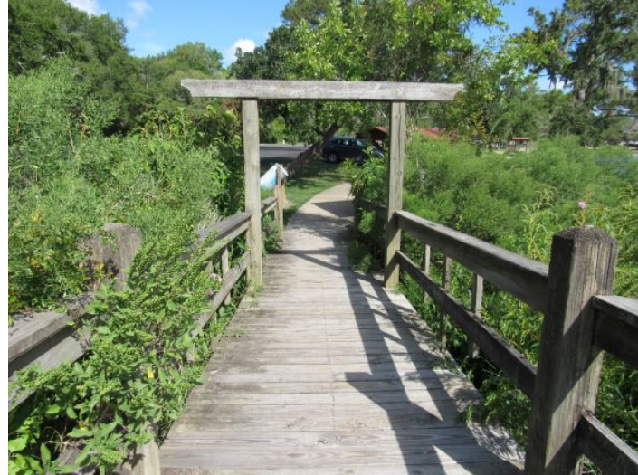
Fishing pier bridge
