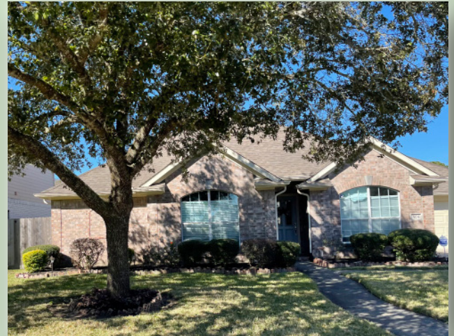
Typical single-family detached residence in the Bayou Park subdivision. Source: Halff Associates
