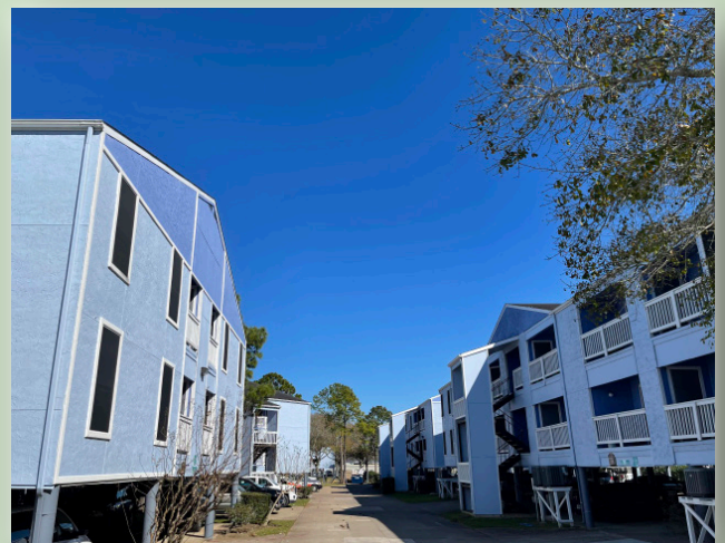
Interior view of Bayou Village Apartments. Source: Halff Associates
