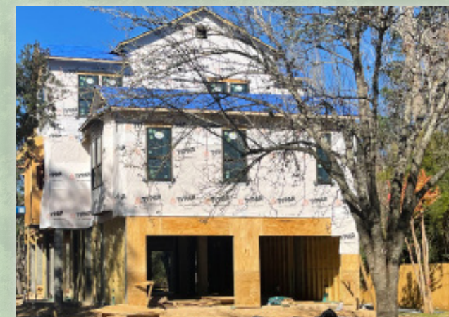
New residential construction on Desel Dr. Source: Halff Associates
