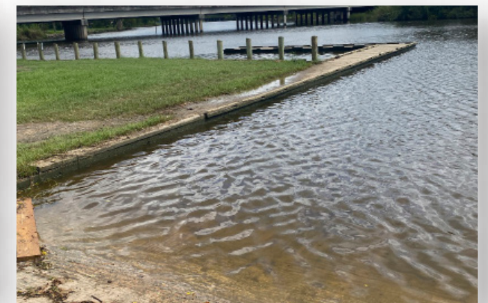
Galveston County's Highway 3 Boat Ramp Source: Halff Associates
